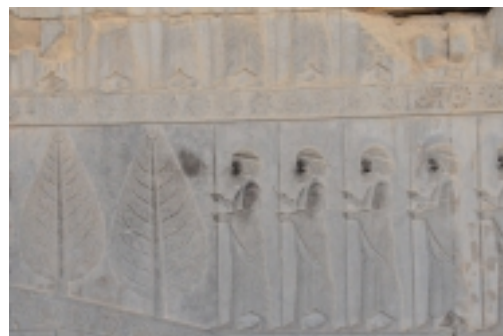
Fig. 1, E staircase of the Apadana Palace: The black colour of the stone is covered by a grayish layer and, in the upper parts of the staircase, by a reddish earthy encrustation
